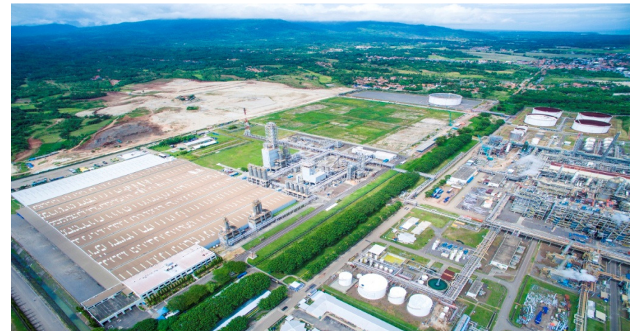
Future SBR Plant Facility Area
