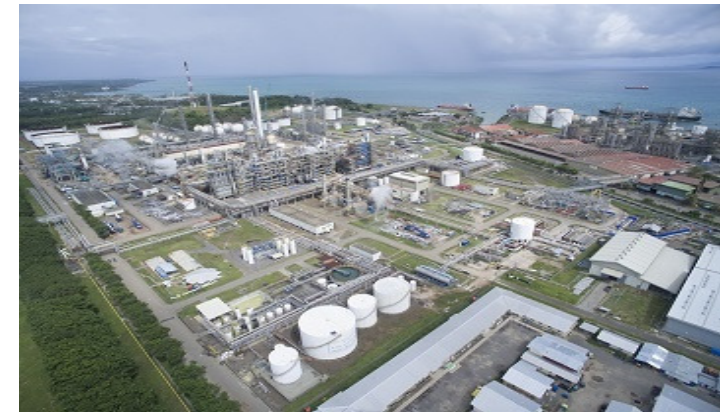
CAP's main integrated manufacturing complex
