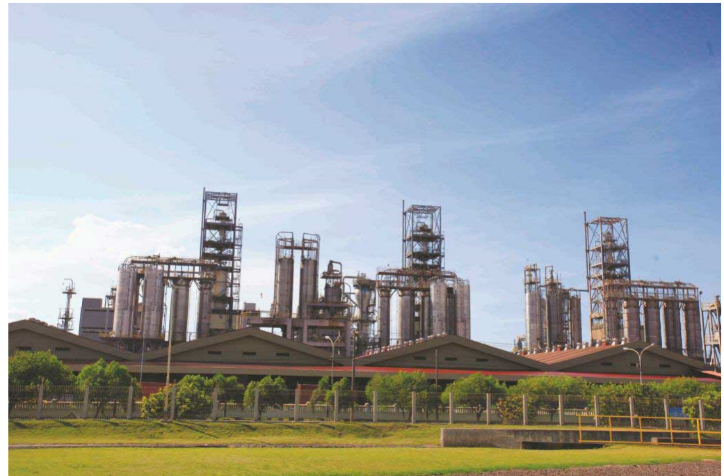
Existing PP plant in Cilegon with capacity 480 KTA, 3 trains of Union Carbide Technology.
